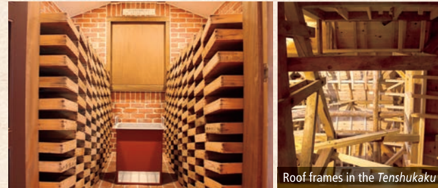
Roof frames in the Tenshukaku
